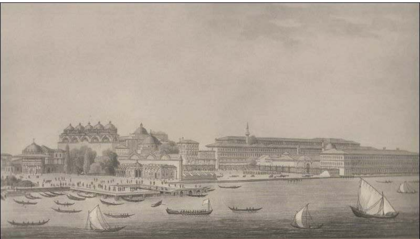
The Topkapi Lock yard
