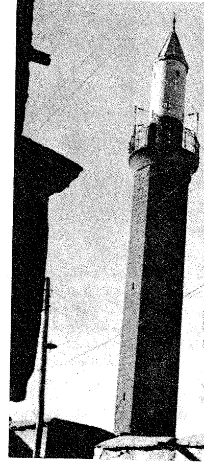
Res. 138 — Hoca Ahmed Camii minaresi
